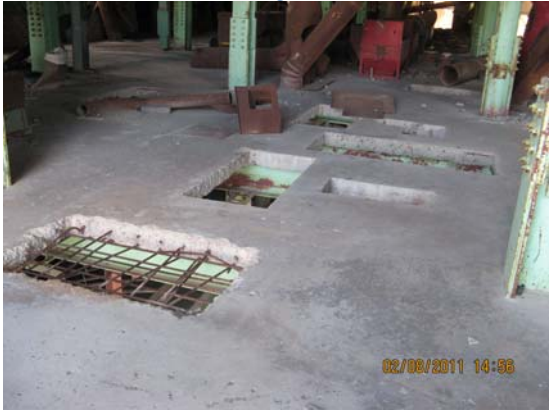
Inside the mill building
